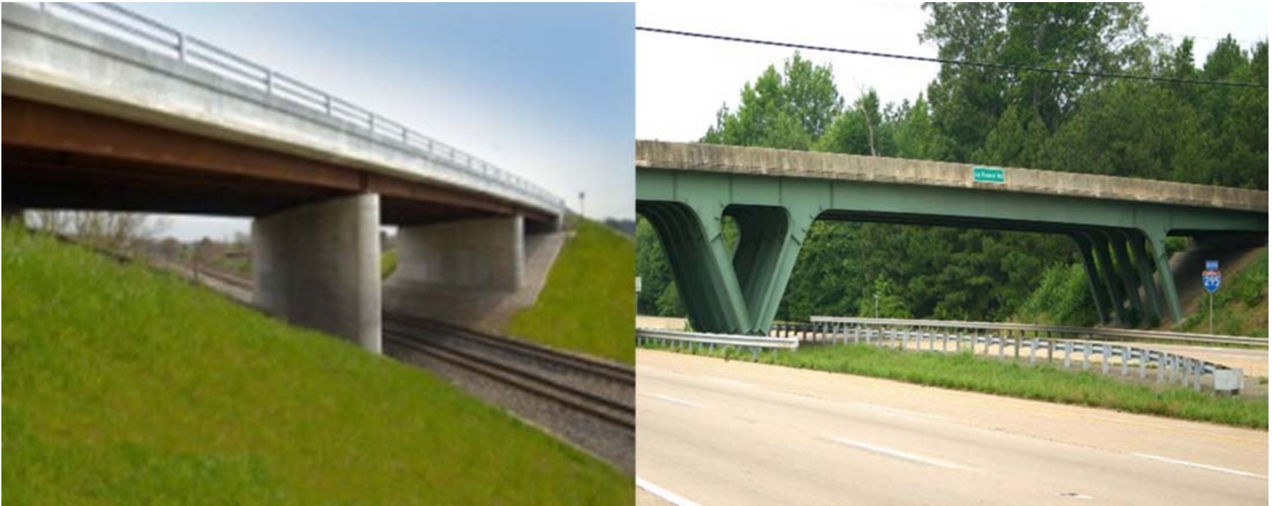
Typical Overpasses Depicting Original 2:1 Slope Design
