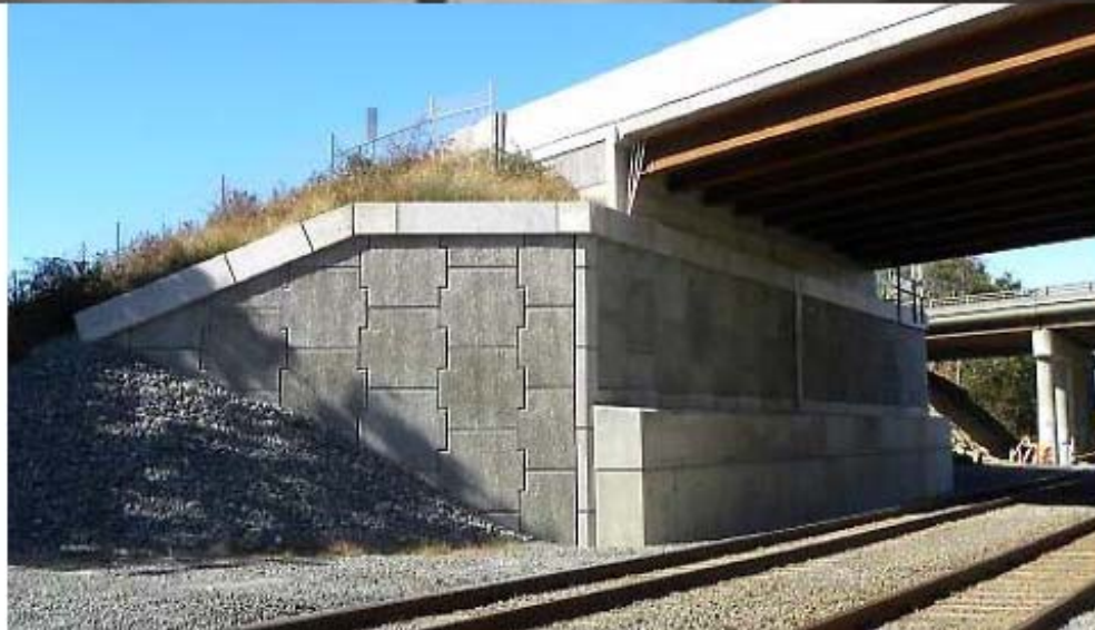
Typical Overpasses Depicting Recommended MSE Wall Design
